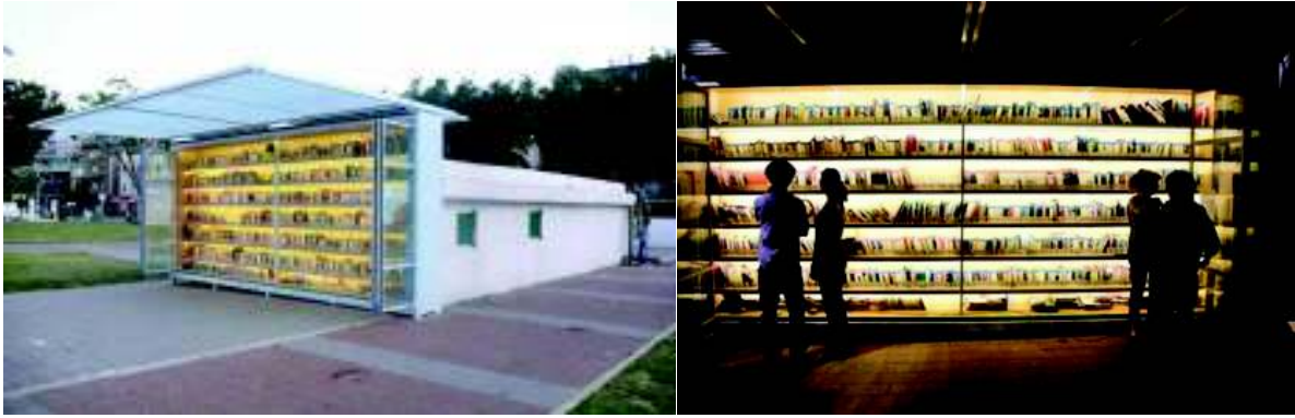
The Garden Library for Refugees and Migrant Workers door Yoav Meiri Architects
